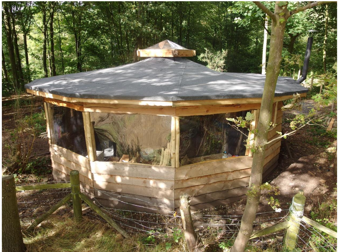
14 th August 2018 - building complete, hours before I catch a ferry to Ireland!
