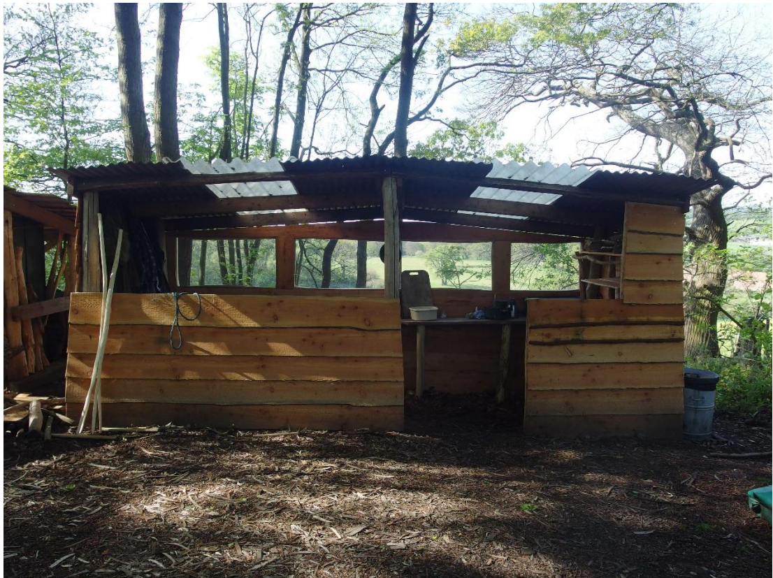
...and the woodland kitchen is renovated.
