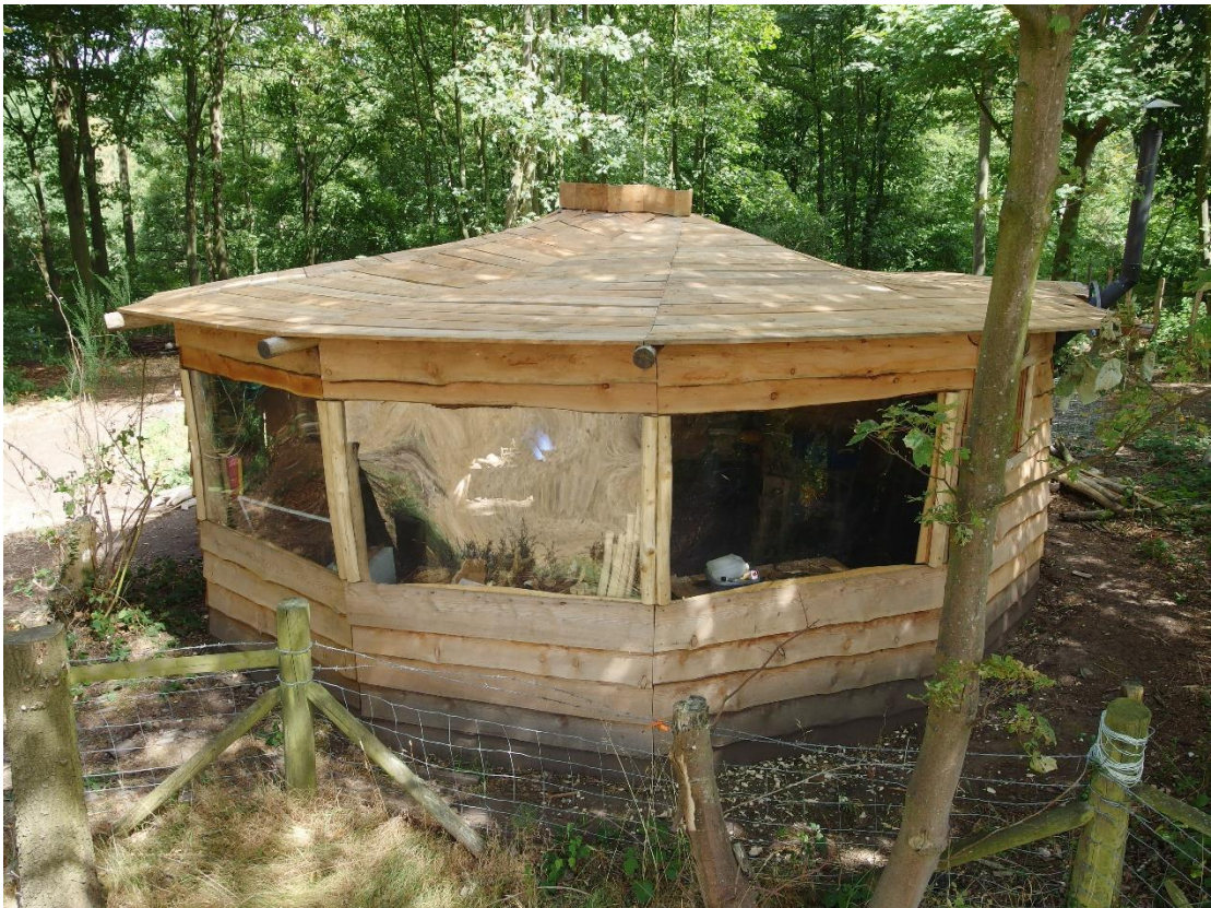
...and centre-piece fitted
