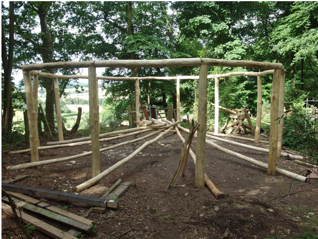
7 th July 2017 - floor-level reciprocal roof trial
