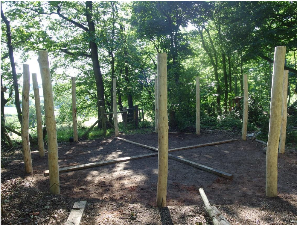
17 th June 2017 - site levelled and all twelve uprights in place
