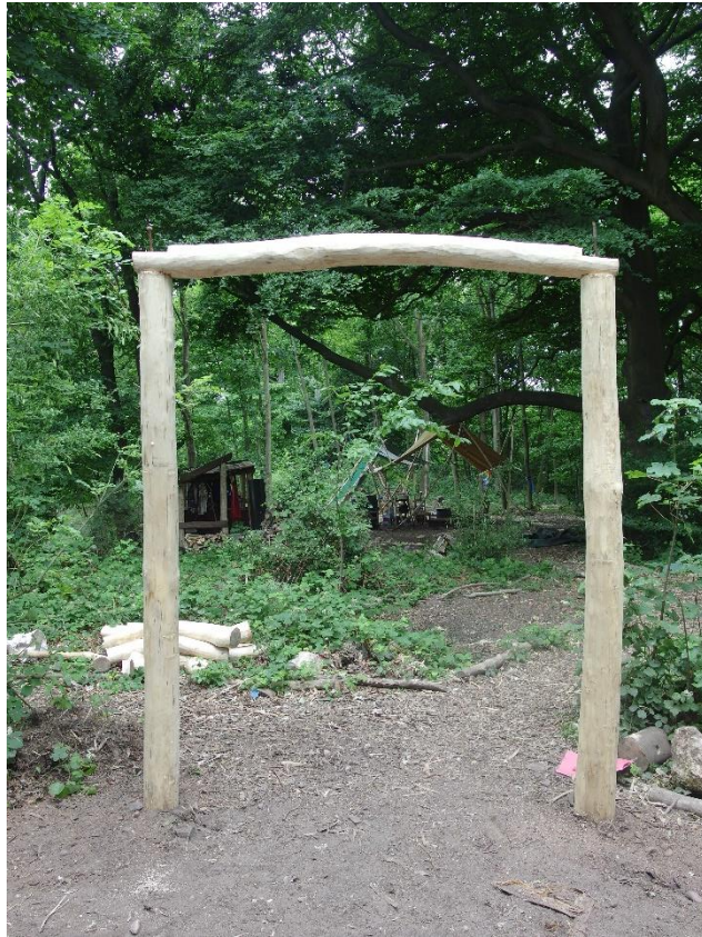
26 th June 2017 - fitting the first tie-beams to uprights...
