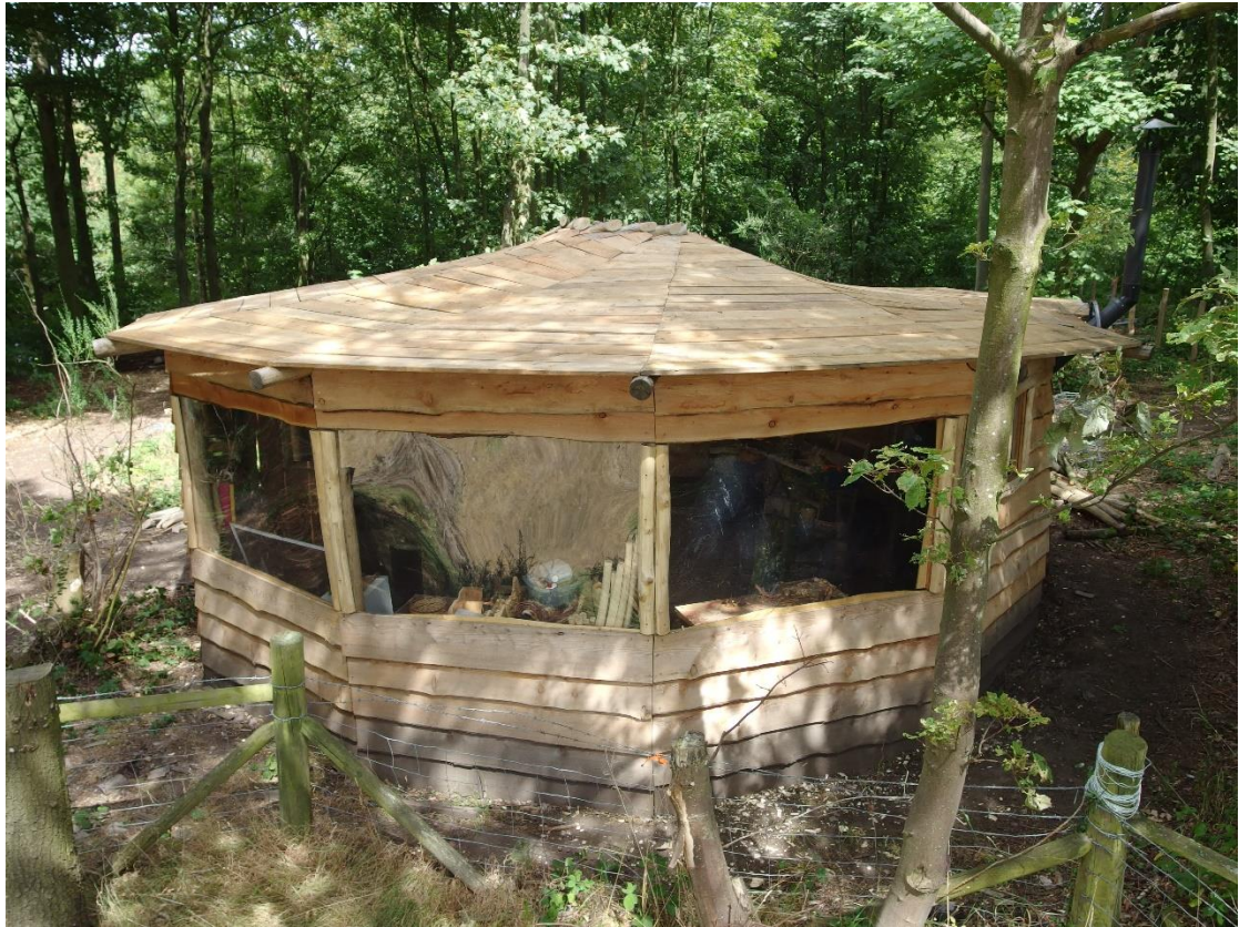
4 th August 2018 - roof cladding complete, chimney in place...
