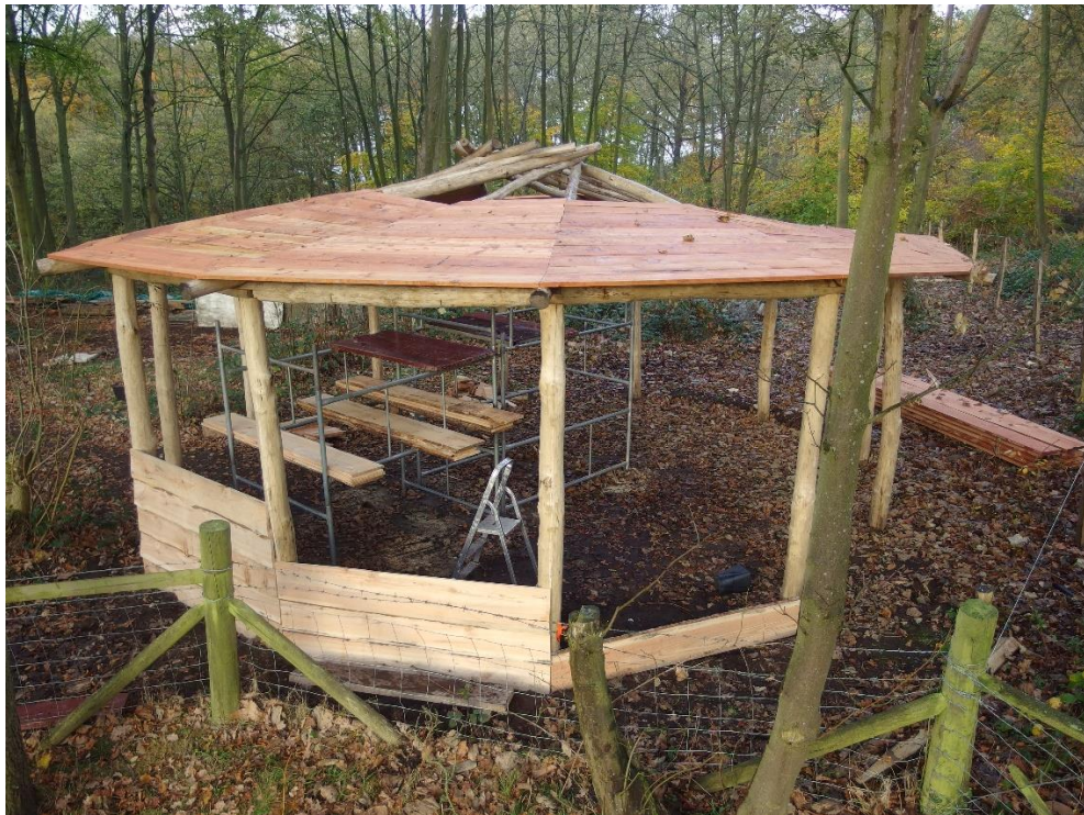
9 th November 2017 - cladding develops...
