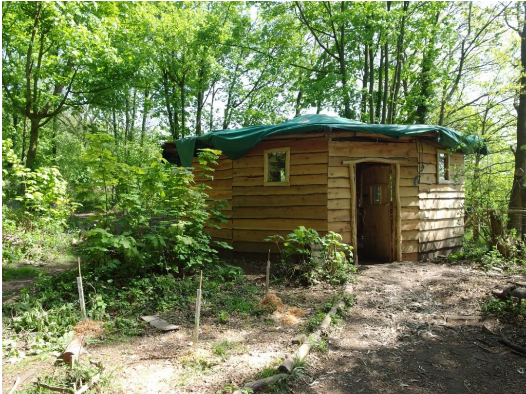
7 th May 2018 - door and all windows fitted, along with a temporary tarpaulin, after a long cold winter
