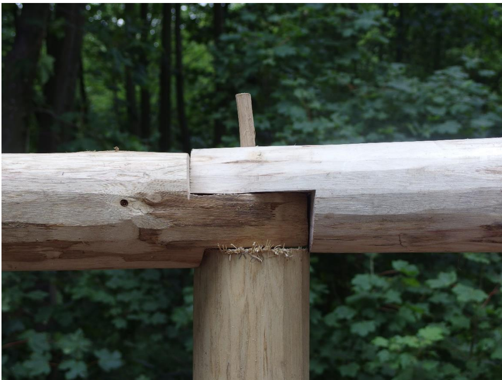
...and securing them in place with a 'lap-joint' and an oak peg
