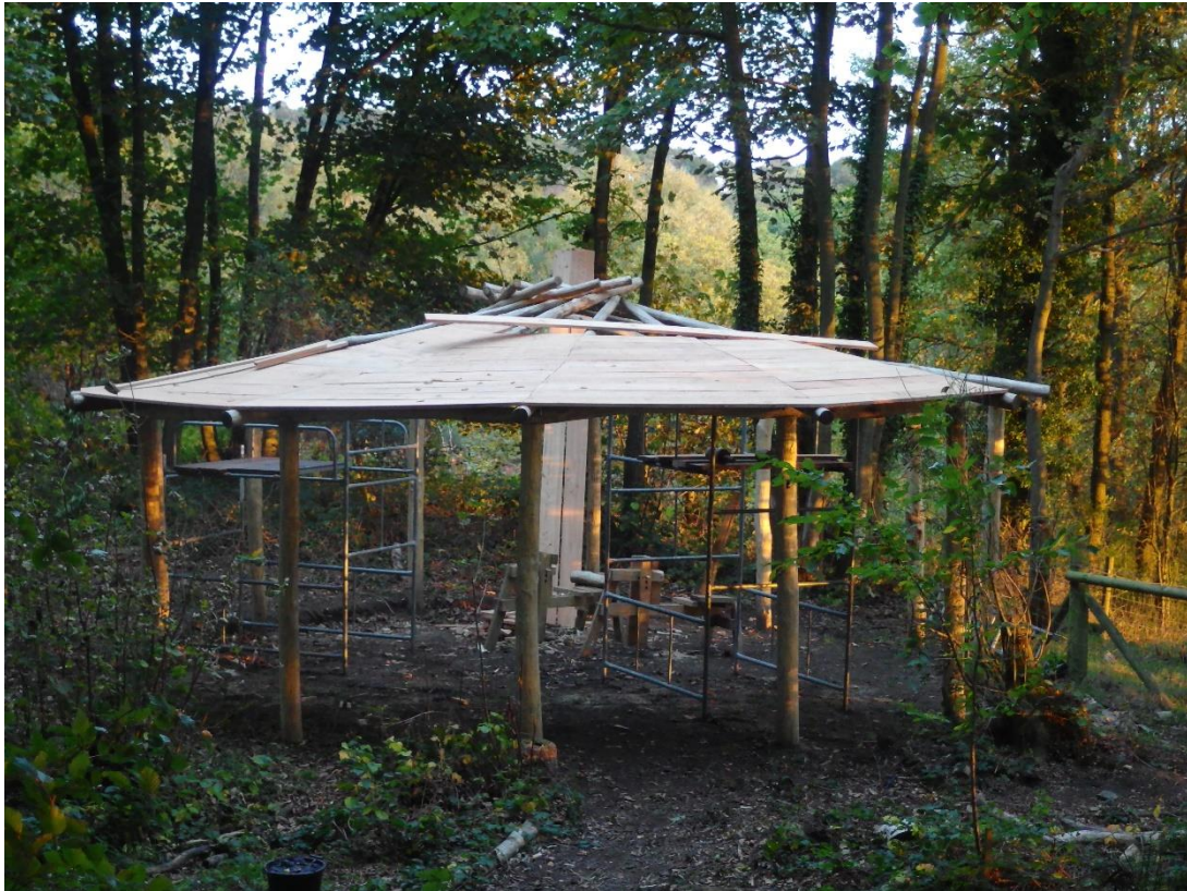
9 th October 2017 - roofing begins...
