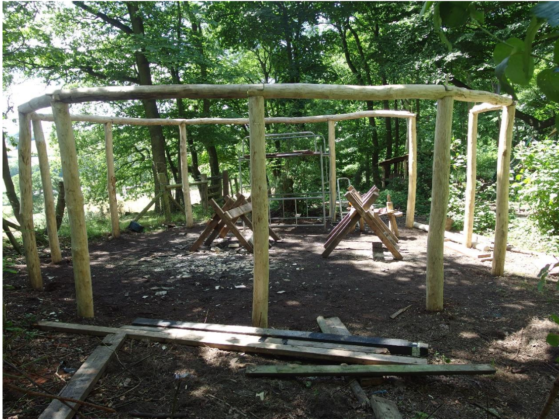
1 st July 2017 - the initial 'henge' nearing completion
