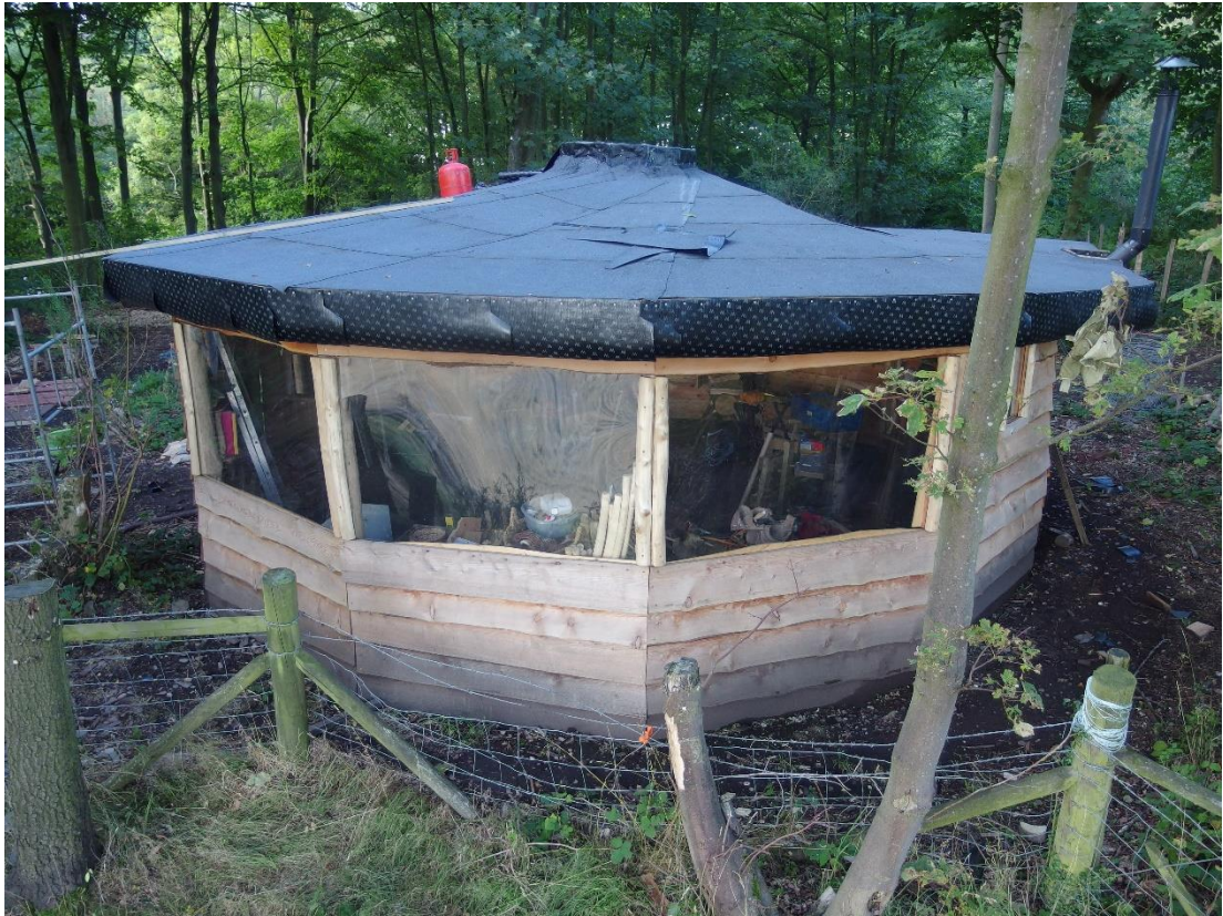
13 th August 2018 - final layer of felt in situ
