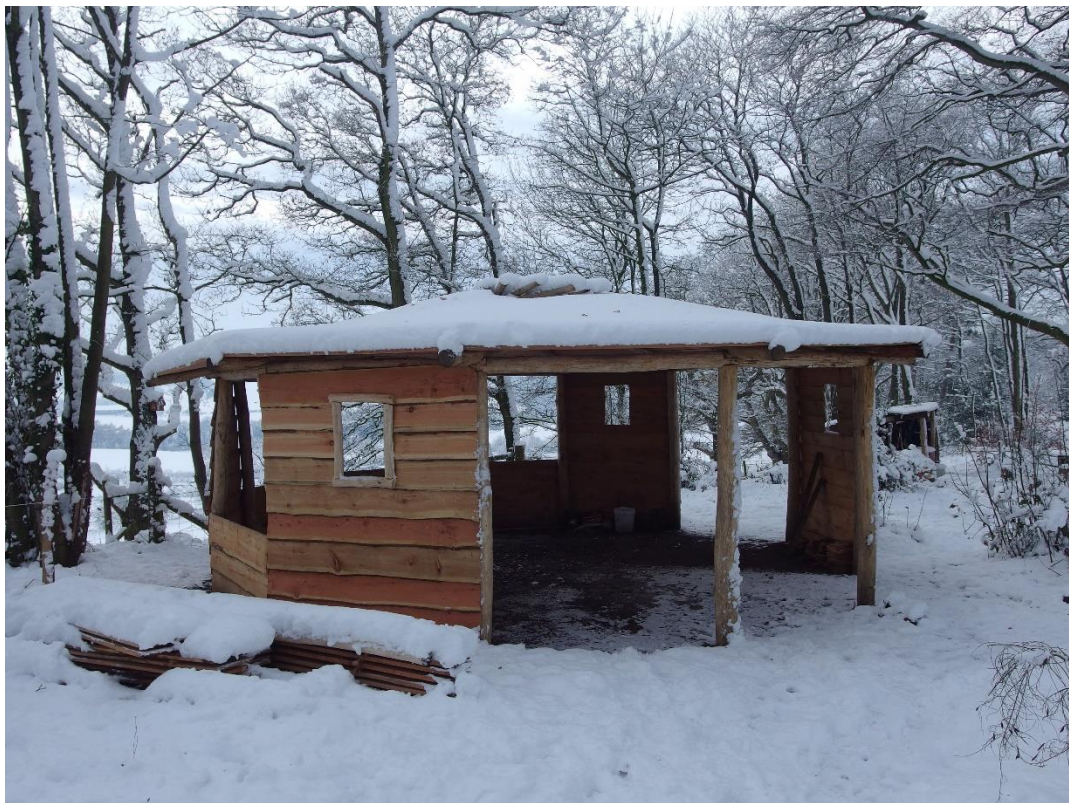
12 th December 2017 - the roof holds up despite the snow!
