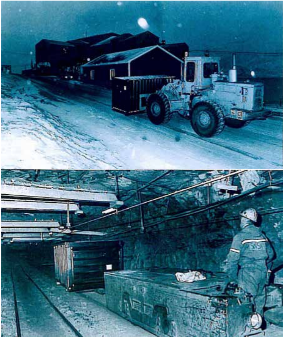
Figure 1. Transport of the steel container from the airport and into the coal mine was carried out by Store Norske Spitsbergen Kulkompani. Images from Hempel Information, Number 7, August 1985. Hempel is the company that provided the long-term corrosion protection of the steel container.
