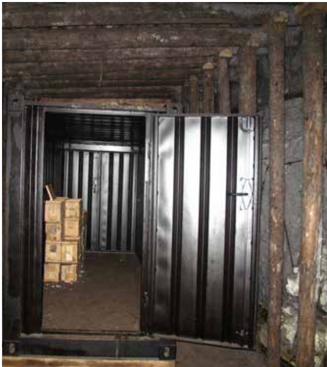
Figure 5. The steel container is placed on a wooden platform in the mine gallery which is strengthened by wood pillars. The photo is taken in February 2017. Only boxes containing seed glass tubes belonging to the 100 year experiment are still stored in the container.
