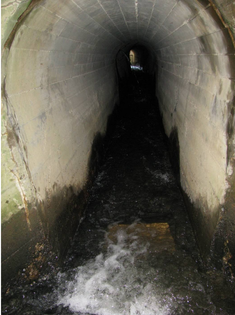
Figure C. Culvert upstream Trondheimsveien (downstream station No2).
