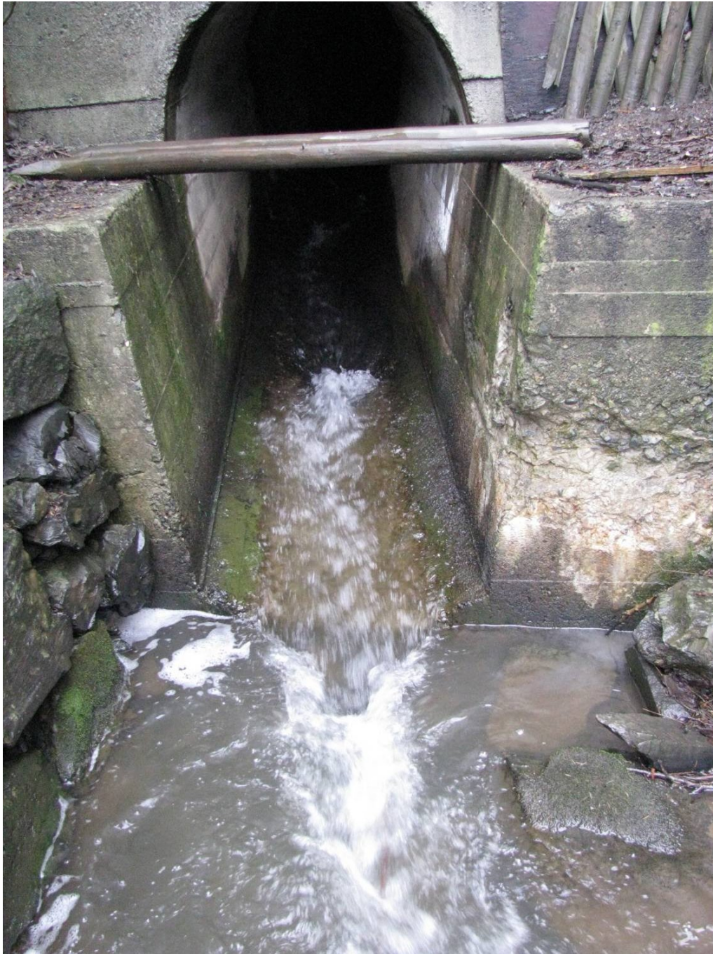
Figure D. Culvert downstream Trondheimsveien (downstream station No2).
