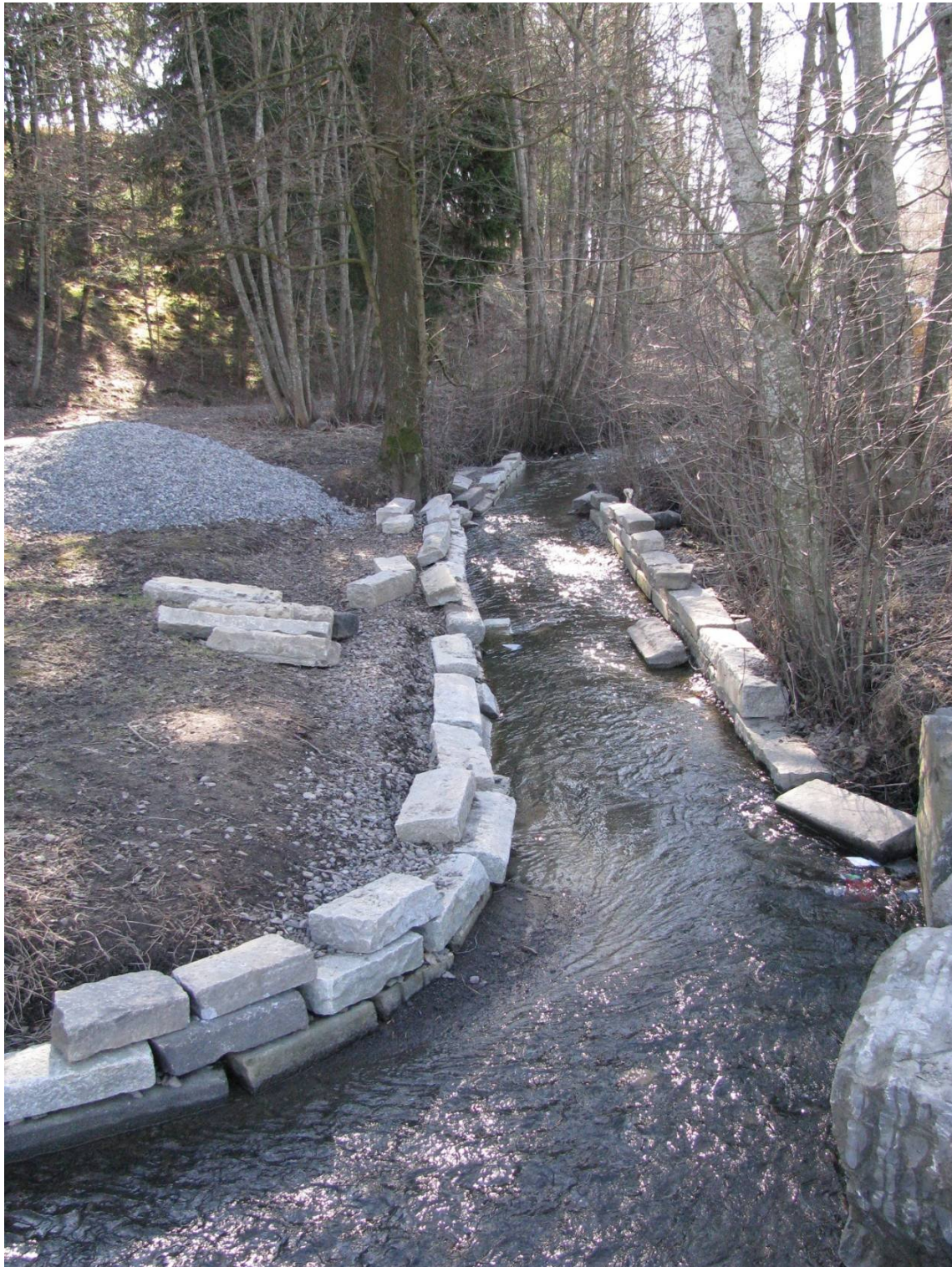
Figure E. Unnatural hardening of the riverbank in station No4.
