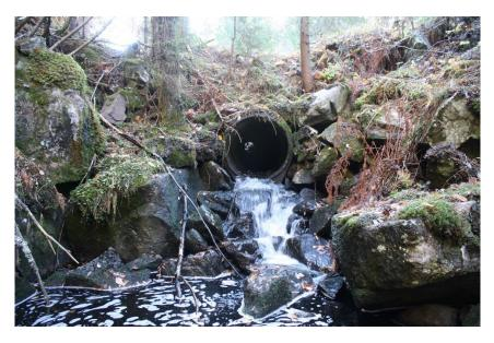
Figure 8: Tributary B, Storrsjøbekken runs through a small pipe under a road. During normal water flow the pipe is possibly an obstacle for brown trout.
